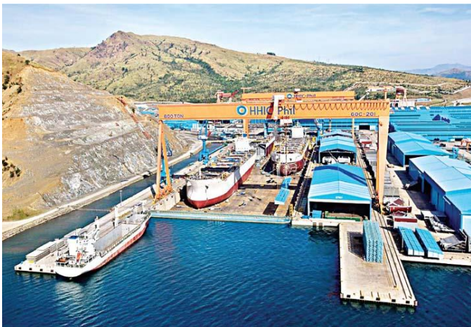
Overview of the shipbuilder Hanjin Heavy Industries and Construction-Philippines (HHIC-Phil) shipyard in Subic Freeport. (MB file photo)
